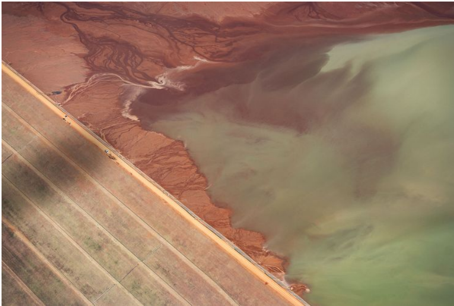
Tailings dam. Photographer: Júlia Pontés for Bloomberg Businessweek
